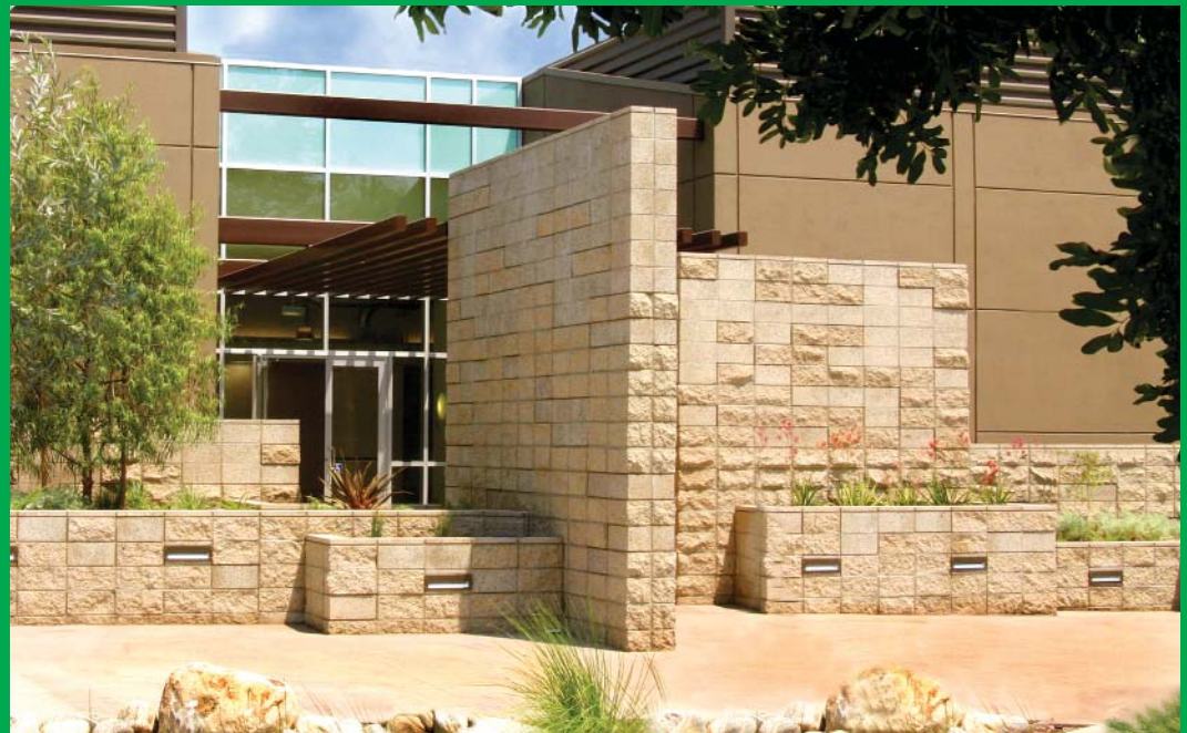
Pacific Oaks' new building at 45 Eureka Street, Pasadena.
